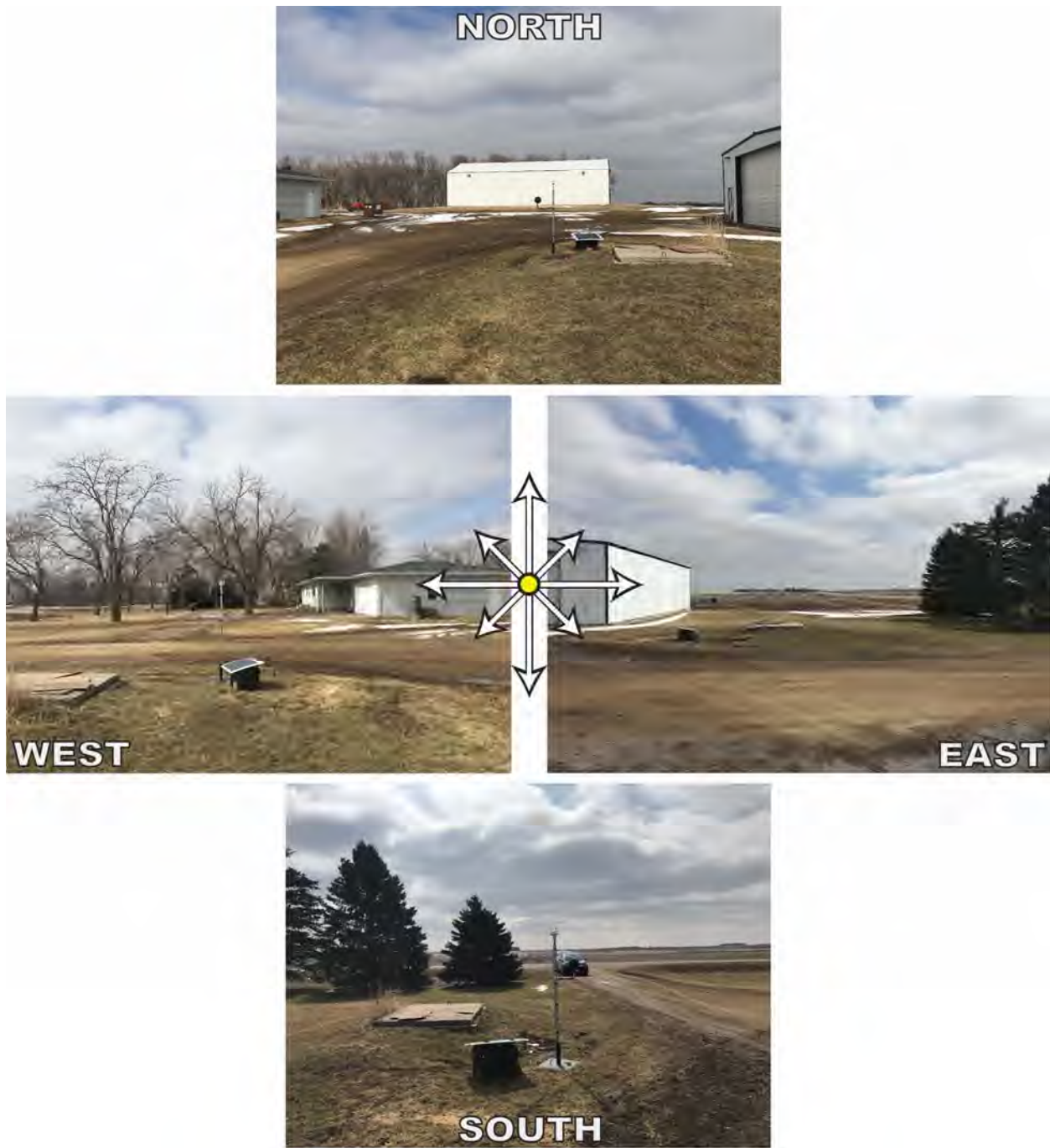
Figure A-1. Measurement Location M1 Photographs
