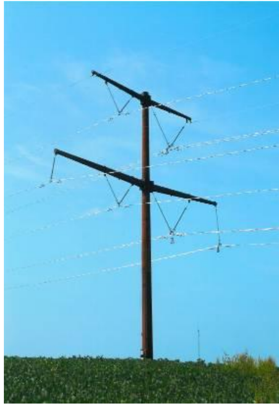
345 kV/161 kV Low Profile Double-Circuit
