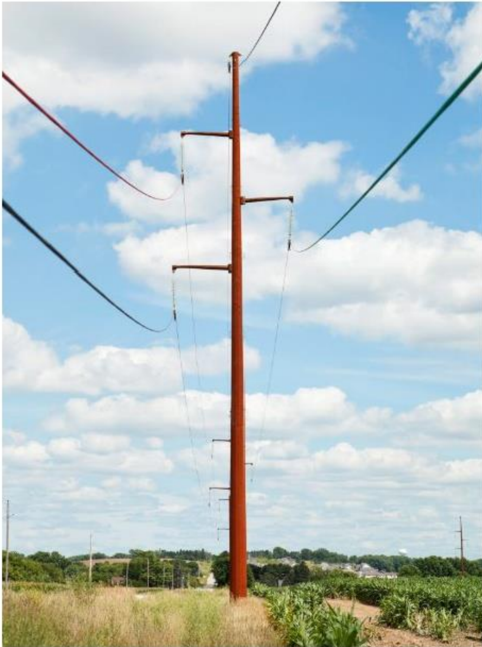
Figure 3-2 Photograph of Typical 161 kV Transmission Structure
