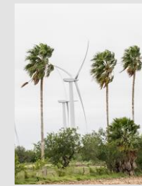
Cameron Wind, Texas 165 MW, 2015
