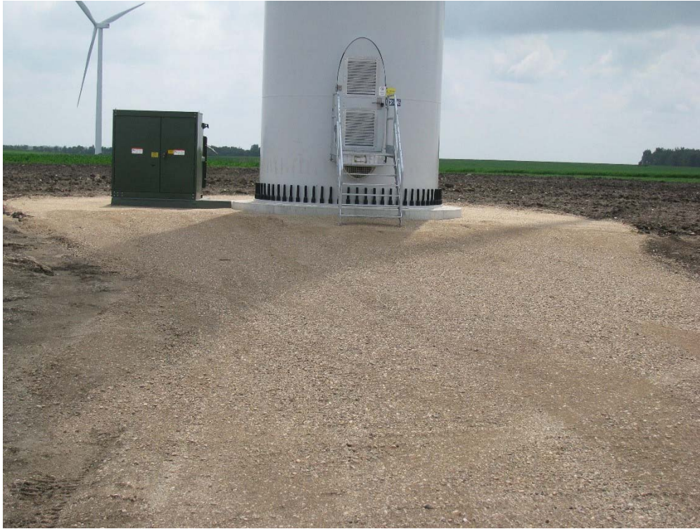
Figure 2: Turbine Permanent Impact Image
