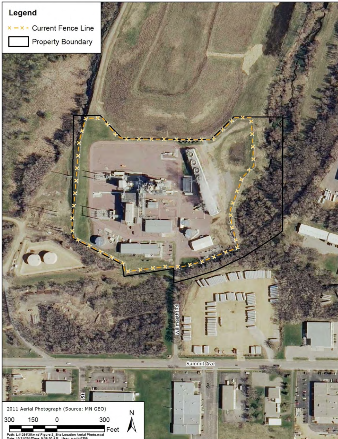
Figure 2. Mankato Energy Center Site
