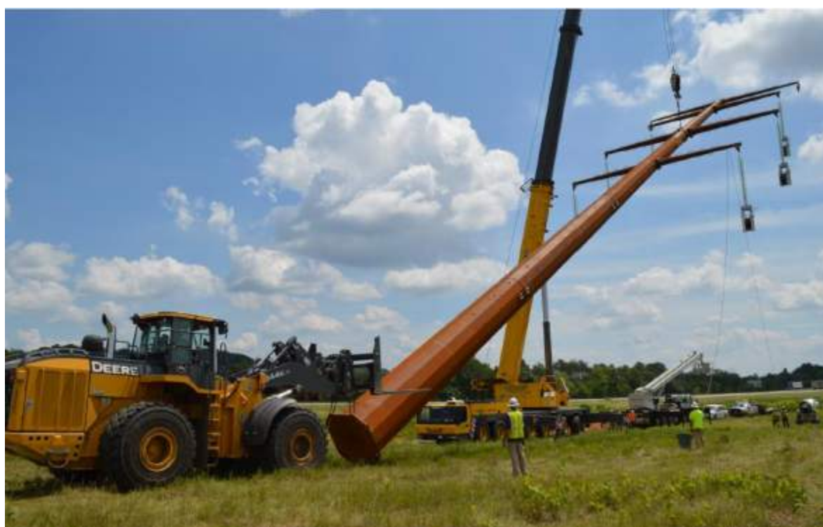
Photo 3-4 Erecting Structure with a Crane
