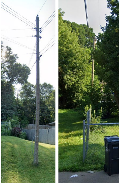
Figure 2-8 Existing Overhead Lines for an Undergrounding Project
