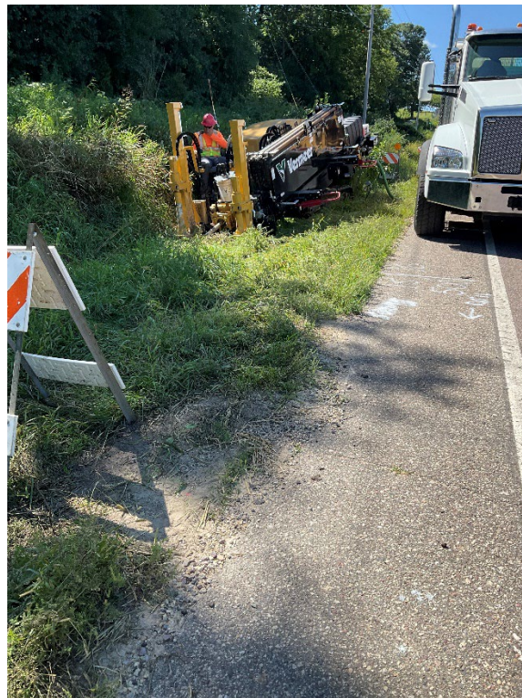
Figure 2-11 Directional Boring Operation Begins
