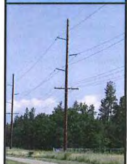
Typical 115 kV Wood Structure with Distribution Underbuild
