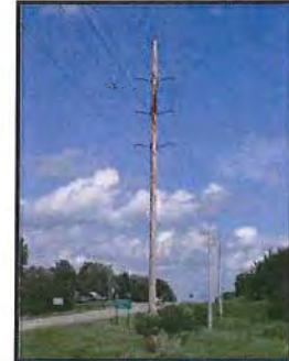
Typical 115 kV Wood Double Circuit Structure
