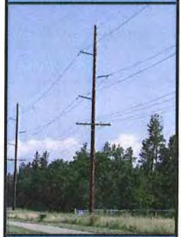
Typical 115 kV Wood Structure with Distribution Underbuild
