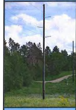
Typical 115 kV Wood Single Circuit Structure
