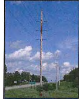
Typical 115 kV Wood Double Circuit Structure
