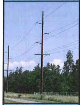
Typical 115 kV Wood Structure with Distribution Underbuild
