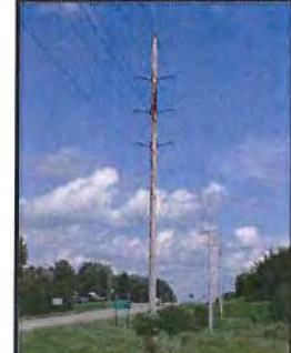
Typical 115 kV Wood Double Circuit Structure
