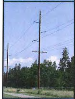
Typical 115 kV Wood Structure with Distribution Underbuild
