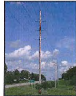
Typical 115 kV Wood Double Circuit Structure
