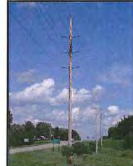
Typical 115 kV Wood Double Circuit Structure
