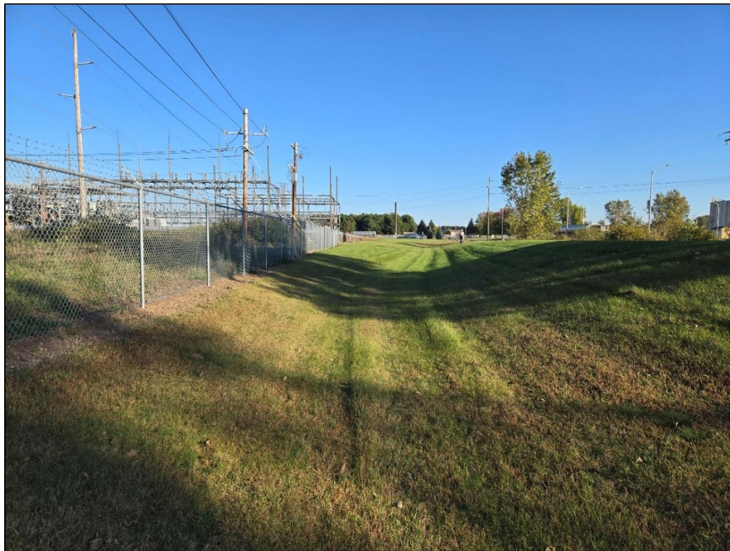
Photo 7. Overview from southwest Property Area, facing north, large drainage area.
