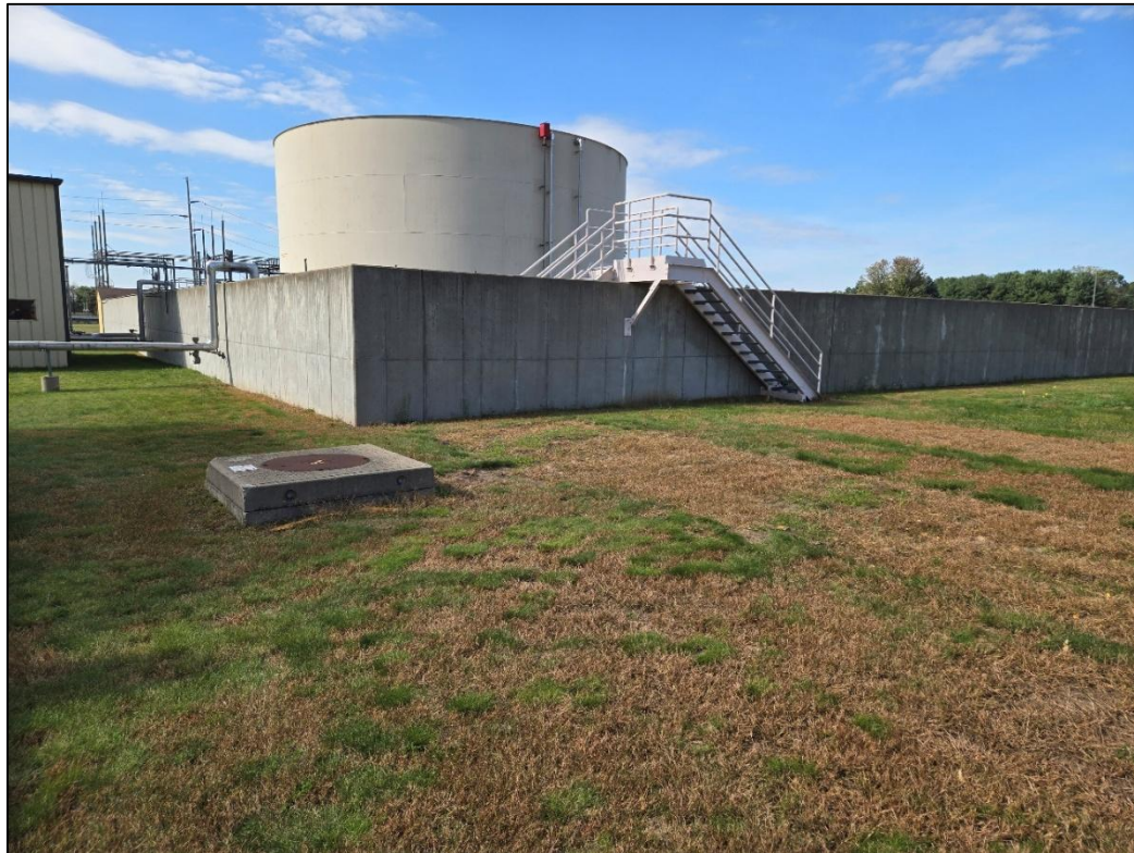
Photo 8. Disturbed area near in place infrastructure.
