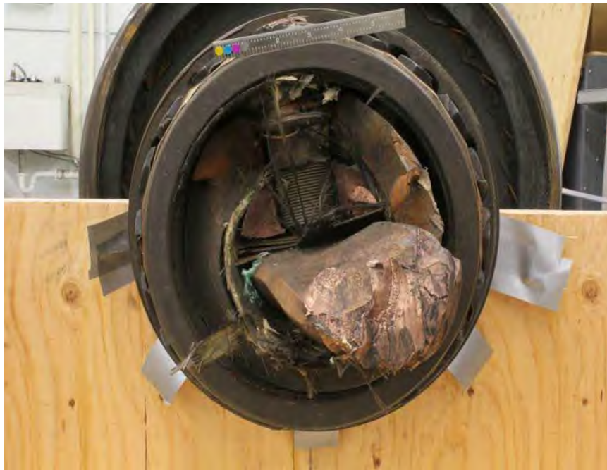
Fig. 310. Aft half of generator shaft fracture.
