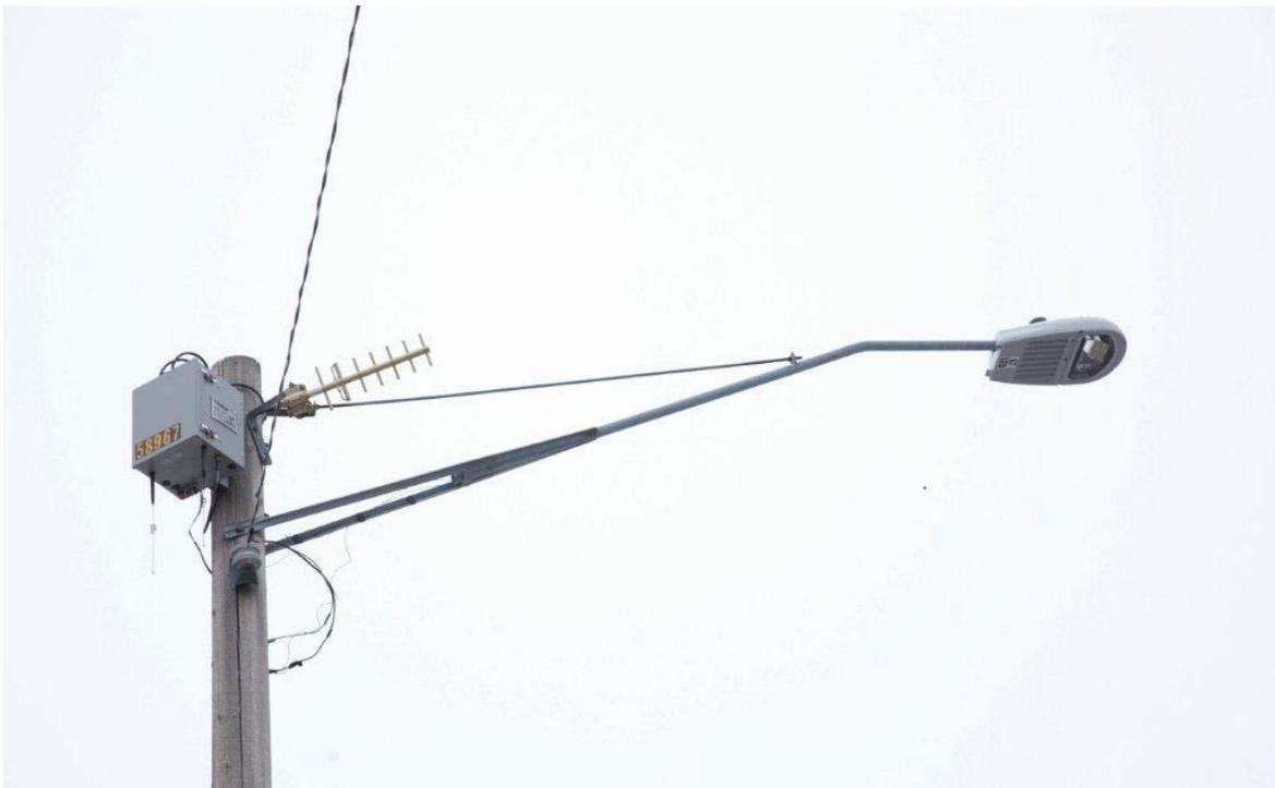
Photo 2: The pilot used General Electric's Evolve™ LED Scalable Cobrahead lighting fixtures.
