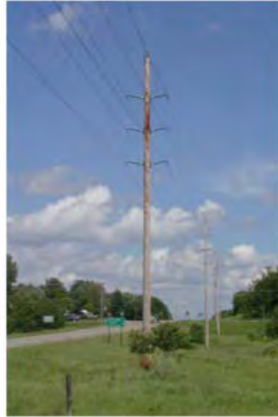
Typical Double Circuit Structure
