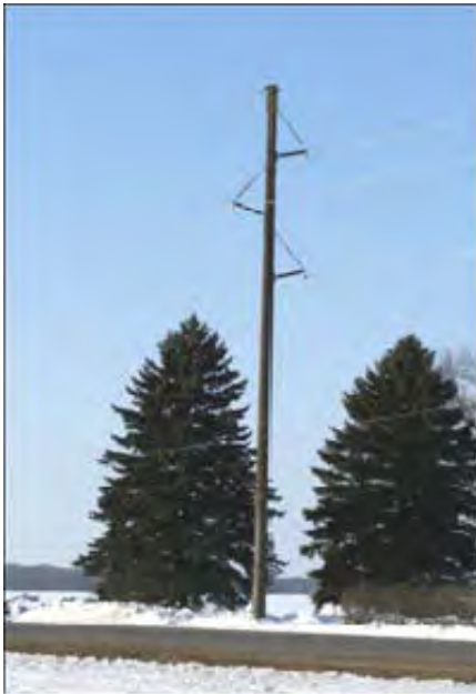
Typical Braced Post Structure
