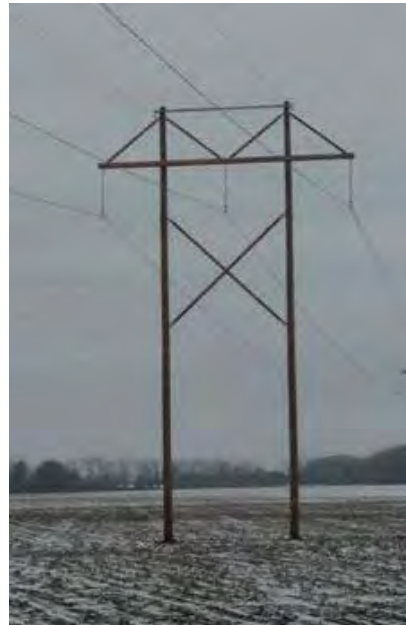
Typical H-Frame Structure
