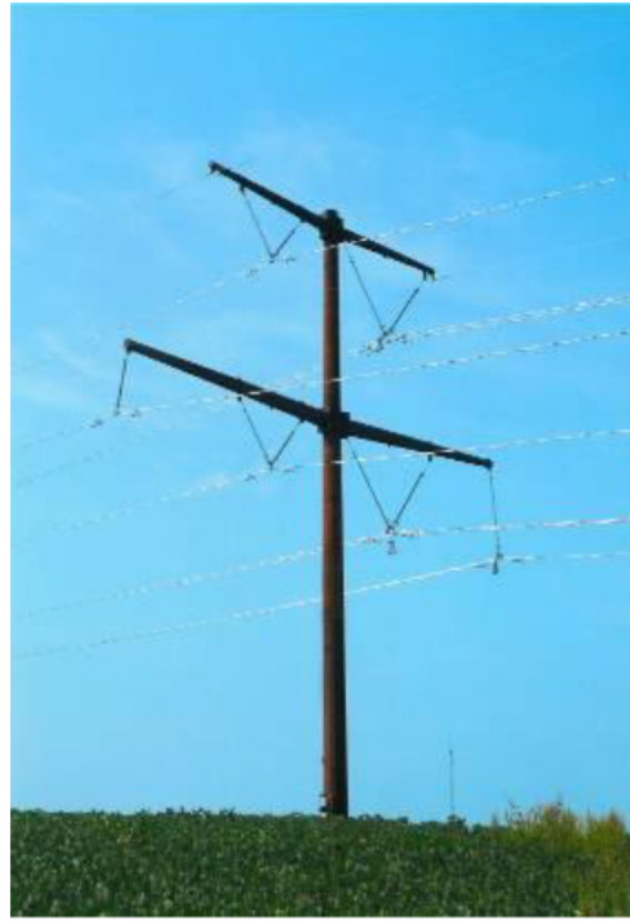
345 kV/161 kV Low Profile Double-Circuit
