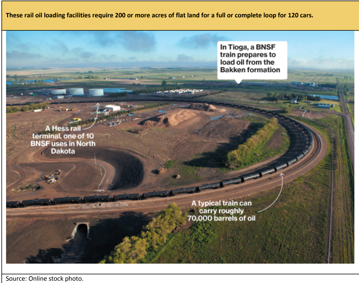
Figure 2-3 A Hess Rail Terminal in North Dakota
