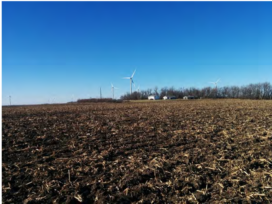
Facing Turbines 50 and 52 from Receptor 37
