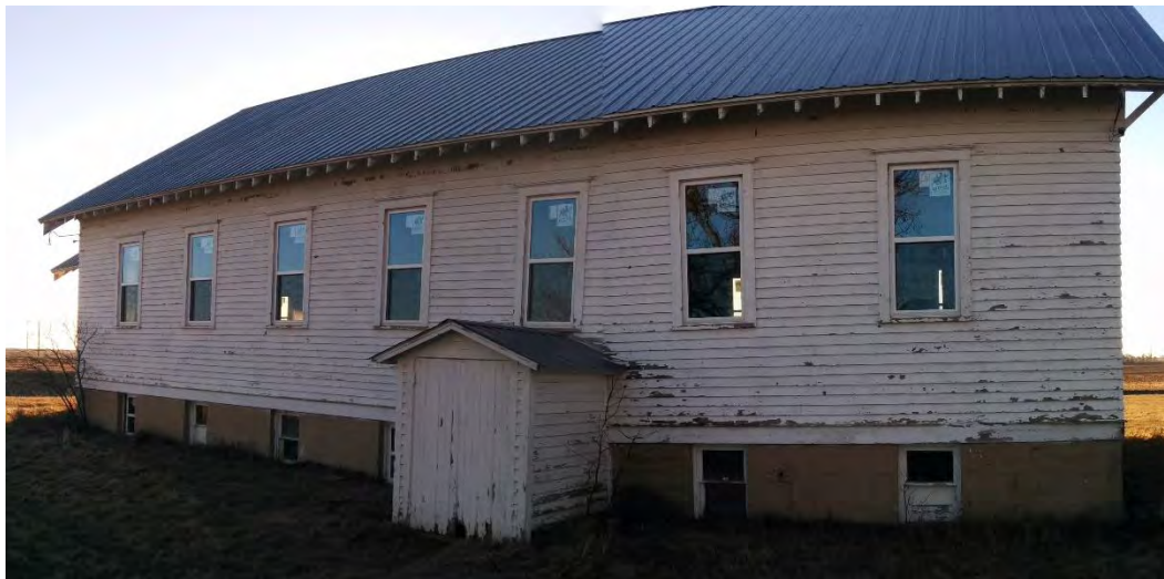
East face of Township Hall
