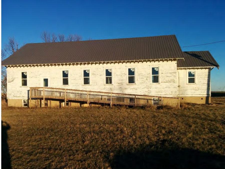
West face of Township Hall
