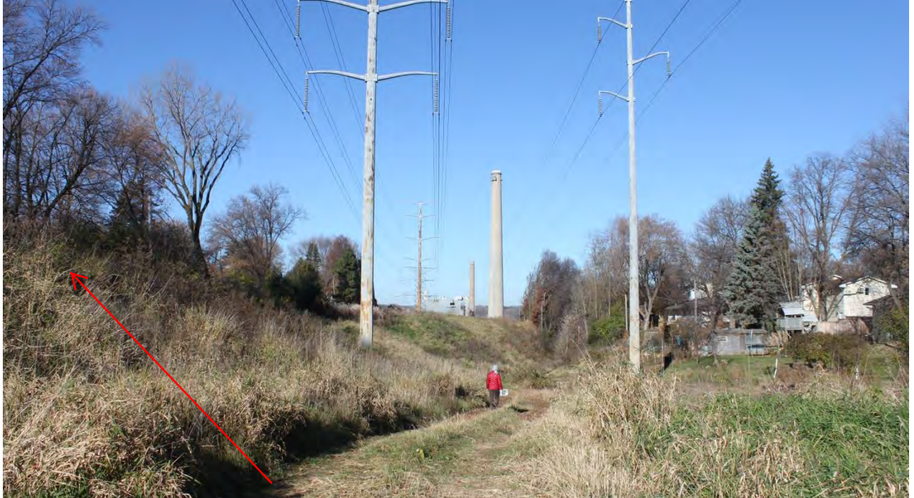
Two-track maintenance road running between existing transmission lines (proposed pipeline alignment is up to the left (NW))
