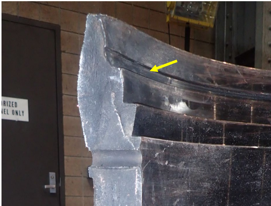
Figure 28. Views of the ID surface profile at the inboard edge the ring (taken at the upper fracture surface (upper image) and lower fracture surface (lower image). The ID slot for the snap ring is indicated by the arrows in each image.
