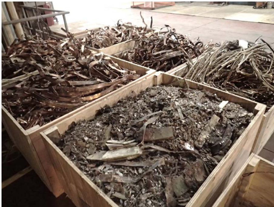
Figure 18. Views of multiple wooden boxes containing fragments of windings and other debris cleaned out of the generator.
