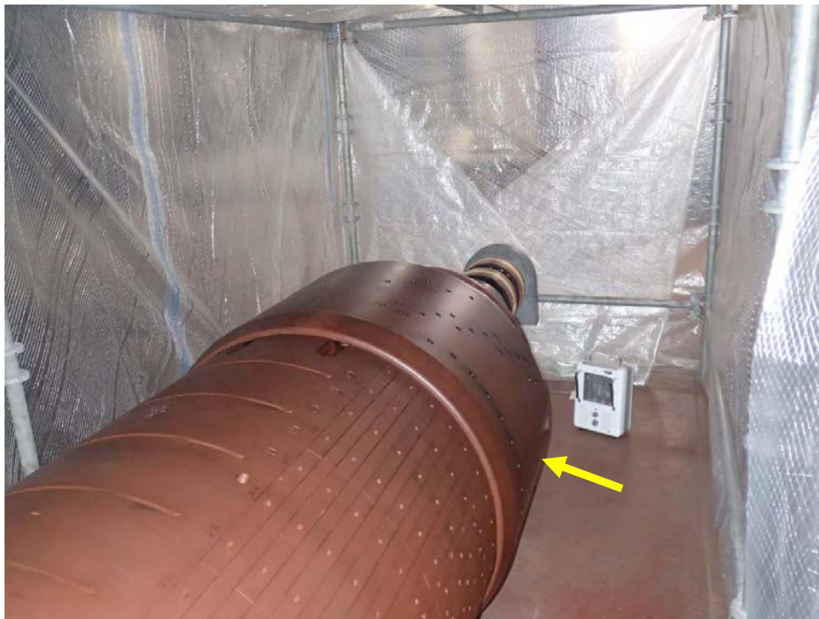
Figure 20. Views of the stored generator rotor, which was tented to maintain a dry storage environment. The lower image shows the intact retaining ring (arrow) at the north (collector) end of the rotor.
