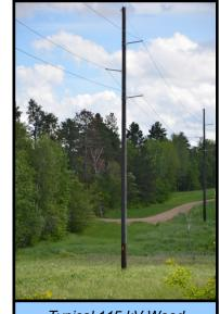
Typical 115 kV Wood Transmission Line Structure
