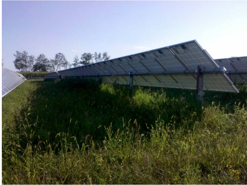
Image 1: Typical Solar Tracker Row Design
