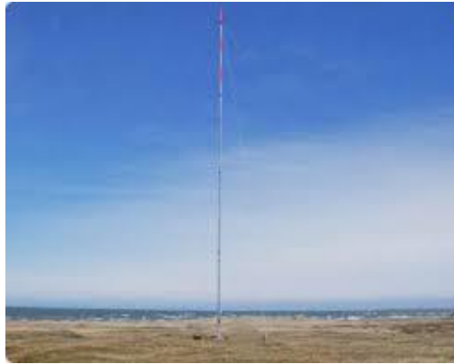
Figure 8. Typical Meteorological Tower 210
