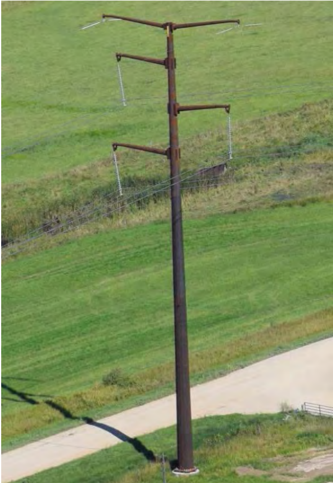
Figure 13: 345 kV Steel Single-Circuit Tangent
