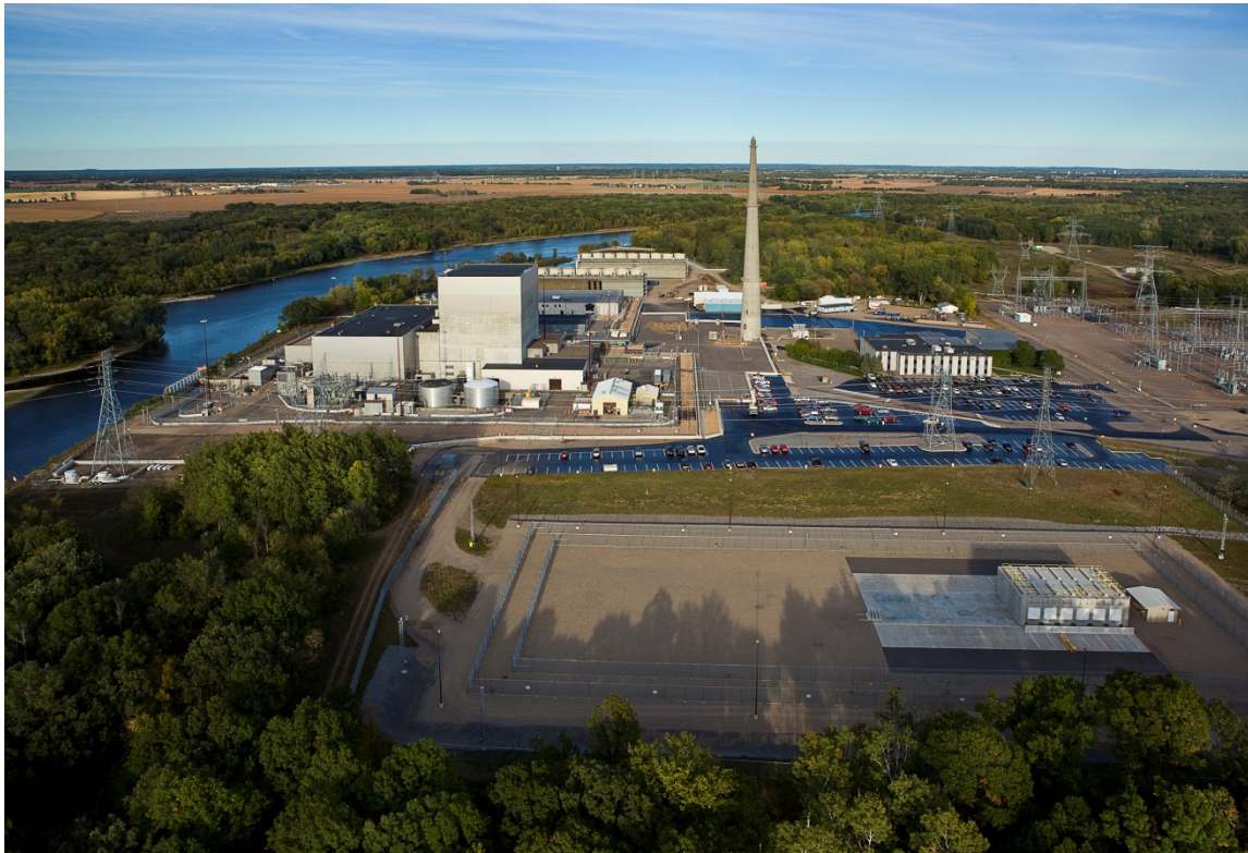
Figure 8-12: Aerial Photo Showing the Dry Spent Fuel Storage Facility
