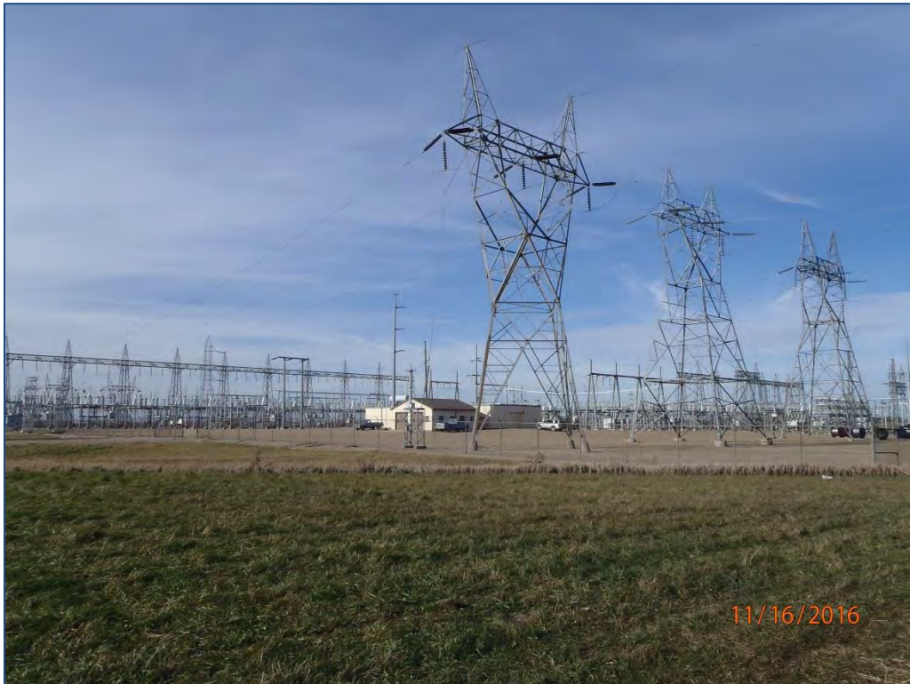
Figure 29. Site 21CP11 overview to the northwest.
