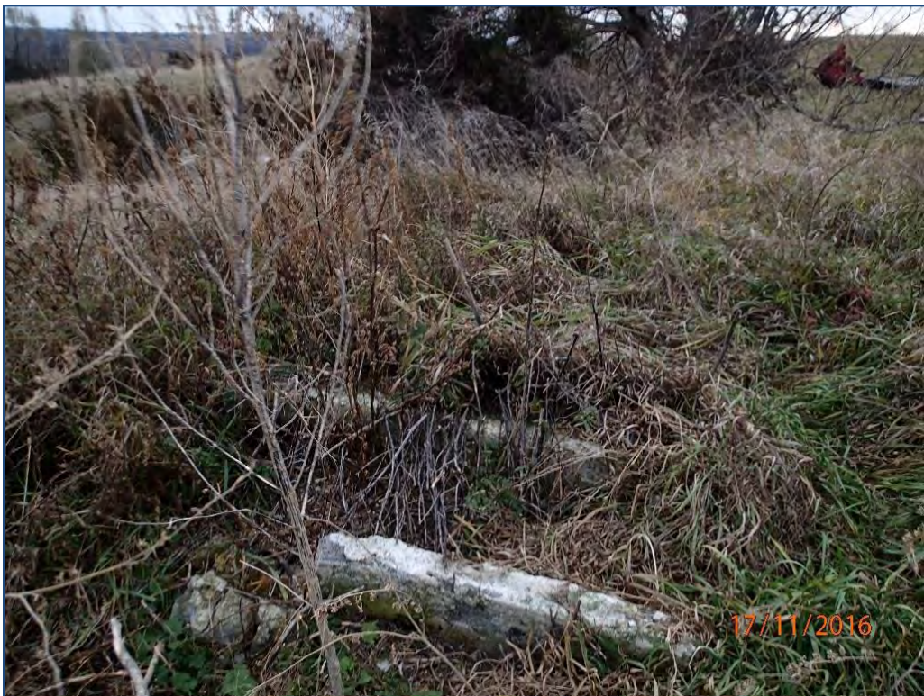
Figure 38. Feature 6: Fragmented foundation view to the west.
