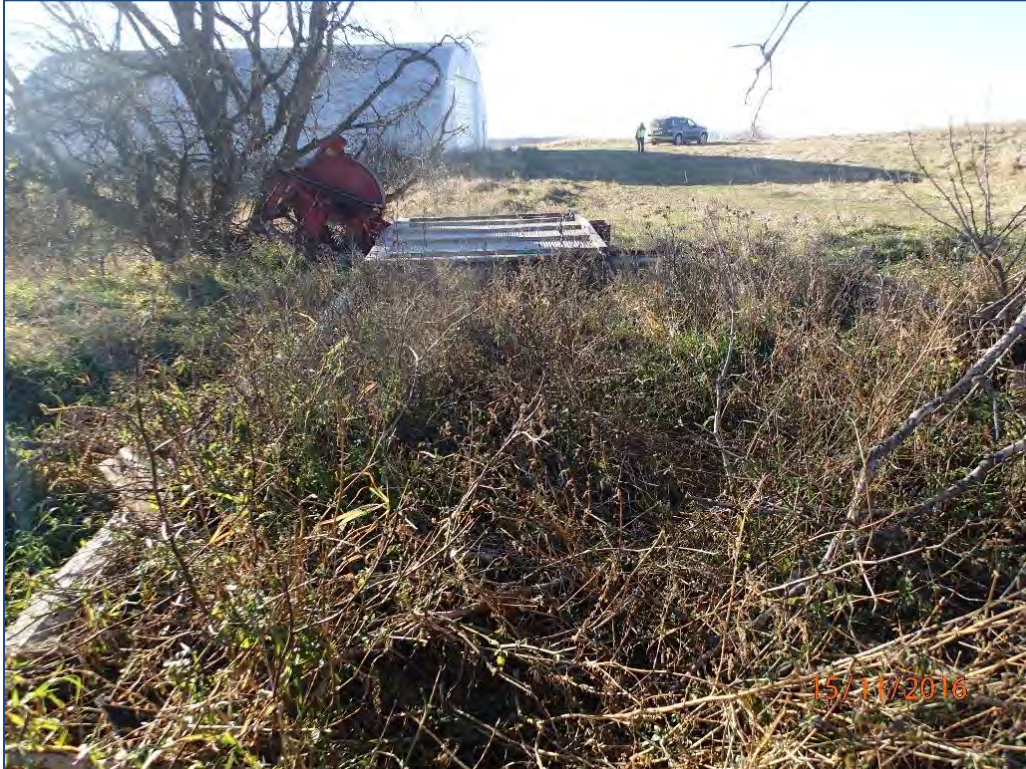
Figure 34. Feature 2: Foundation to the west.
