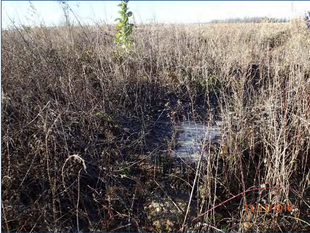
Figure 33. Feature 1: Foundation overview to the north.
