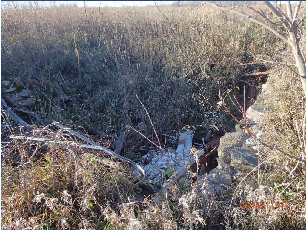
Figure 37. Feature 5: Foundation view to the northwest.
