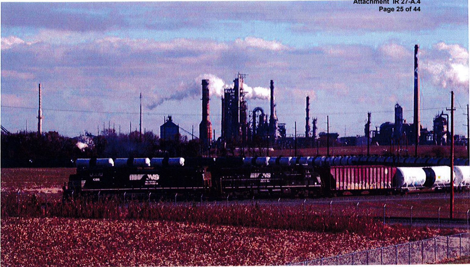
NS oil trains began serving PBF's Delaware City, Del., refinery in 2012. The facility can unload both light and heavy crude oil. Michael S. Murray
