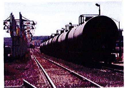
Great Western Railway serves this oil terminal at Windsor, Colo., which in November 2013 was building a two-track platform (left) to load unit trains. Chip Sherman
