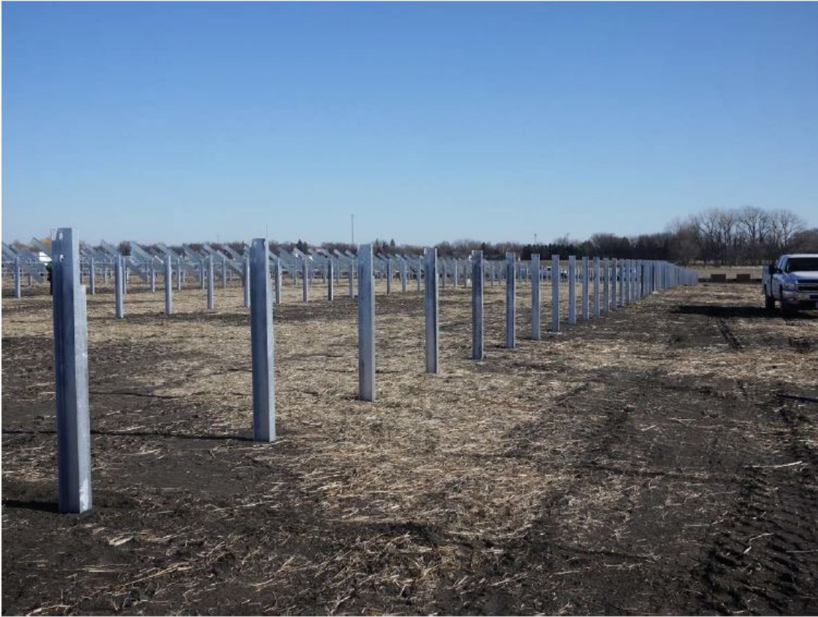
Image 5: Standard Steel Pier Foundations
