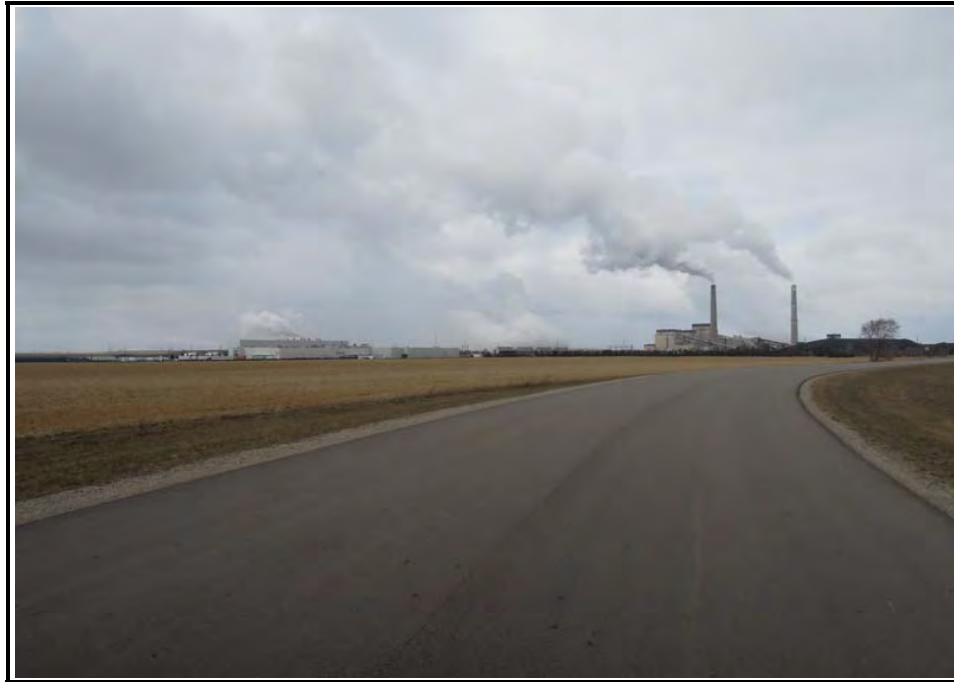
Looking Southwest at Subject from Industrial Boulevard
