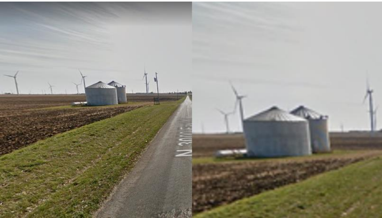
Picture 2: Relative proportions between a turbine and foreground structure from a "close" viewpoint and enlarged image.
