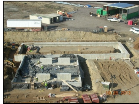
Figure 2: 10-28-2013 Ammonia Unloading/Storage Area/Foundation Work
