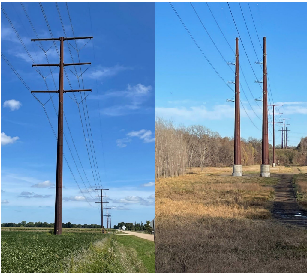
Typical Double Circuit Structures | Typical Dead-end Structures
