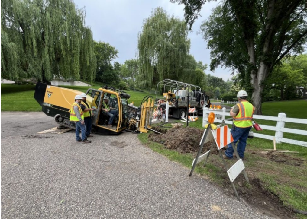
Figure 2-12 Directional Boring Operation Process
