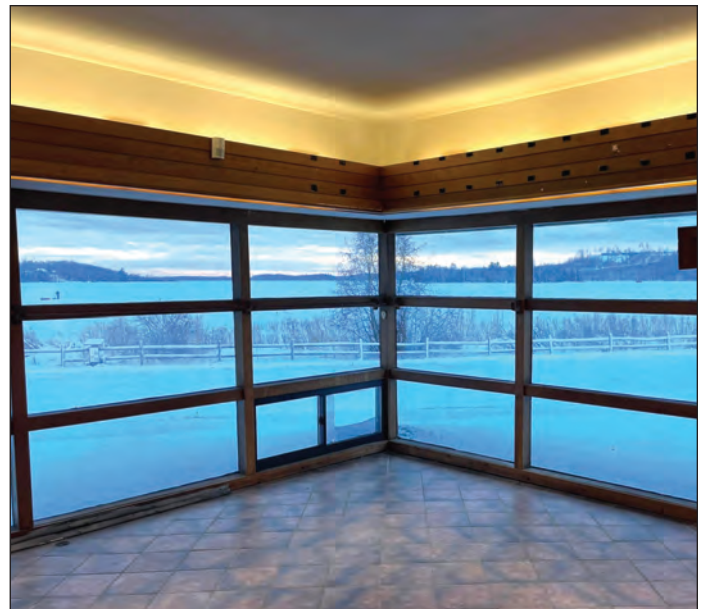
Minnesota Power utility experts offered recommendations for lighting and HVAC updates before the project began.
