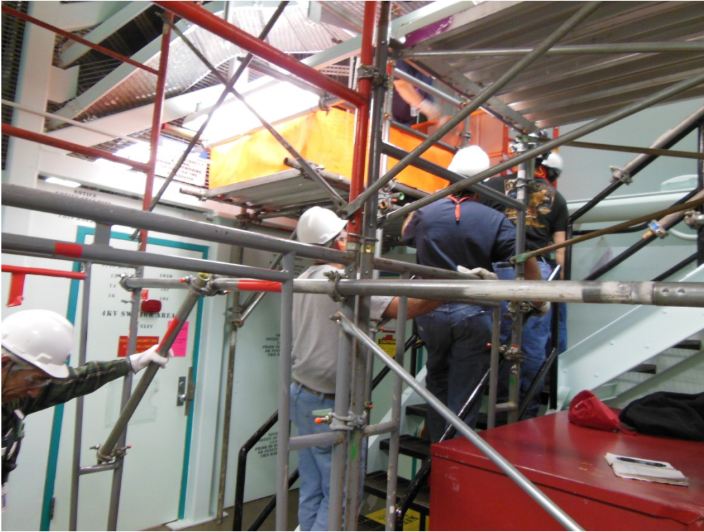
Scaffolding to Area Above 4 kV Equipment for 13.8 kV Conduit Installation
