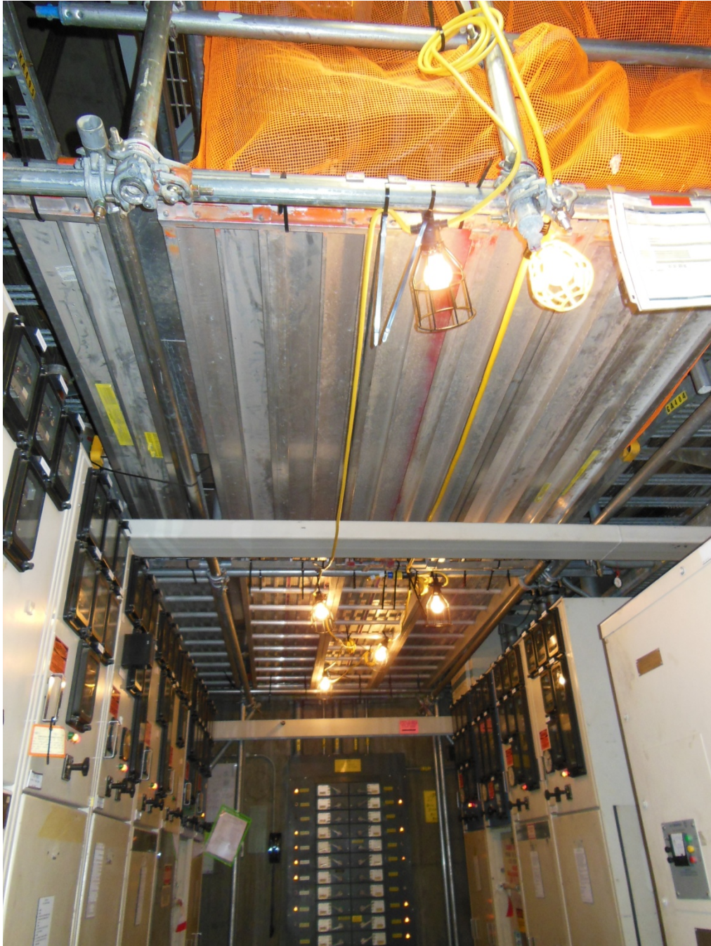
Scaffolding to Protect 4 kV Equipment During 13.8 kV Installation
