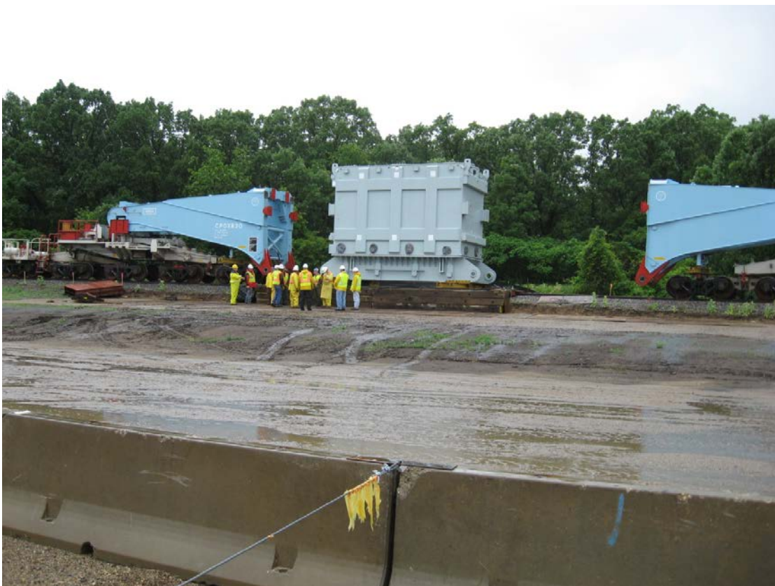
Main Power Transformer Arrival Onsite
