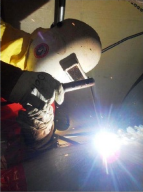
Welding Inside Condensate Demineralizer Vault
