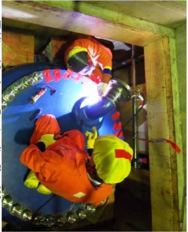
Welding of Condensate Demineralizer Vessel No. 4
