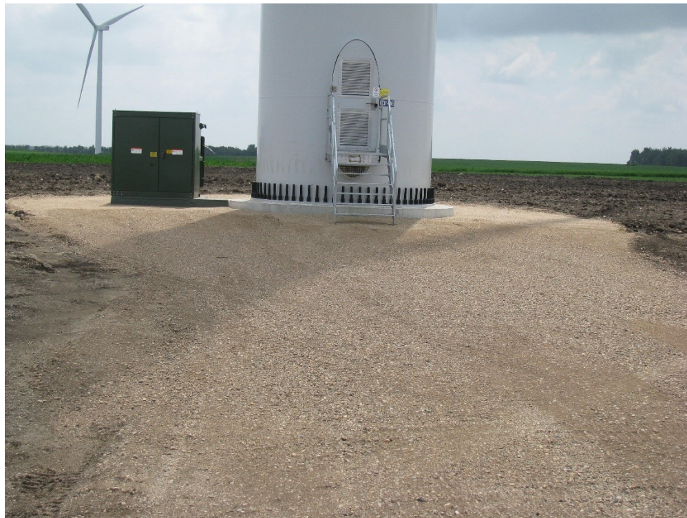
Figure 2: Turbine Permanent Impact Image
