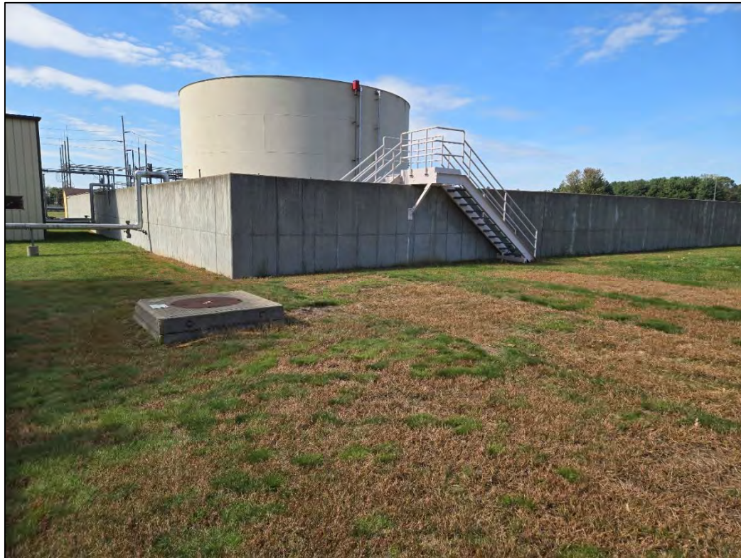
Photo 8. Disturbed area near in place infrastructure.
