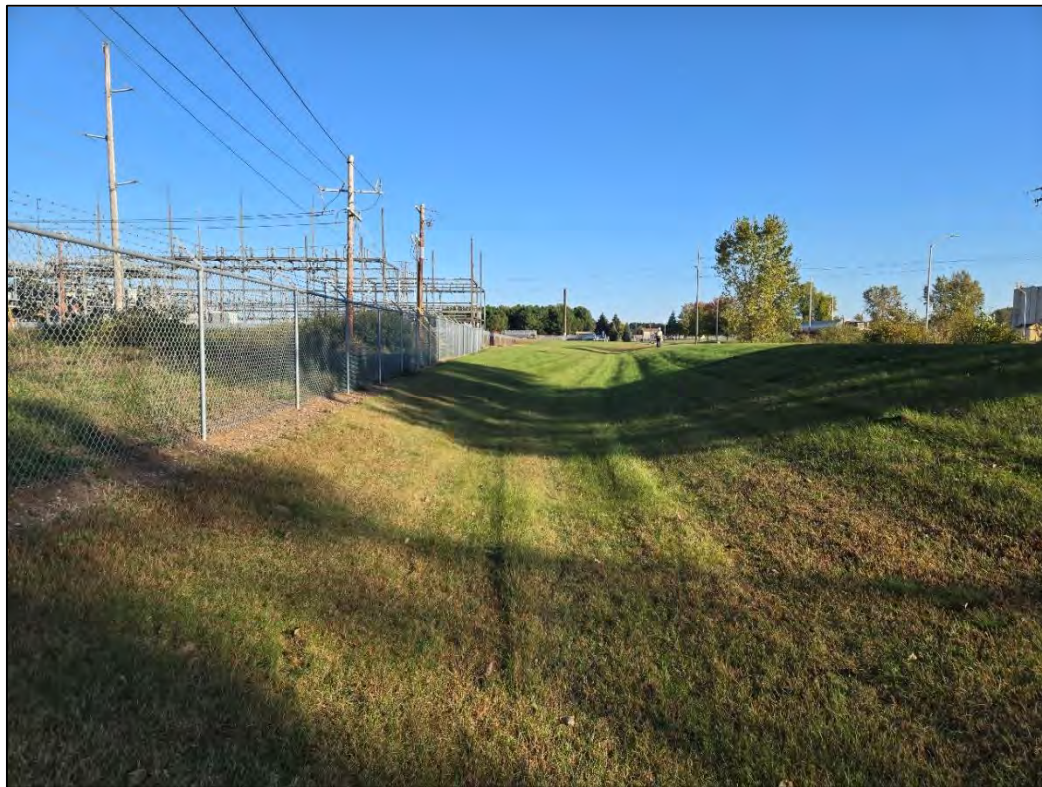
Photo 1. Overview from southwest Property Area, facing north, large drainage area.
