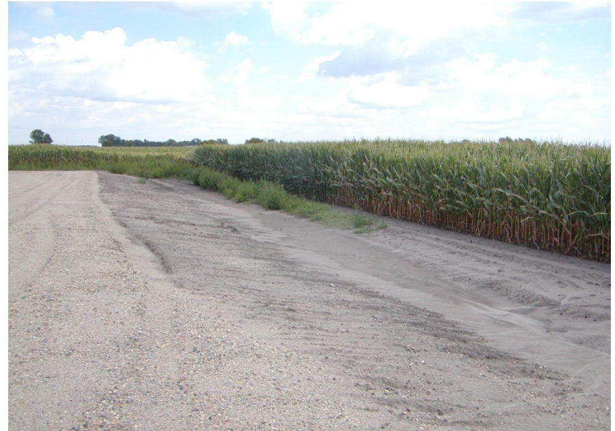
South Edge of Substation Pad: Southwest Corner Looking East
