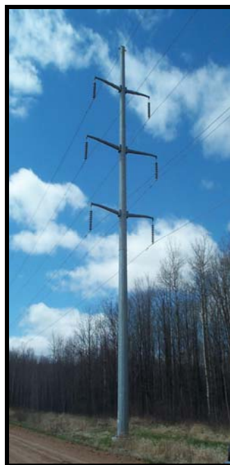
Typical proposed 115/115 kV double circuit structure.
