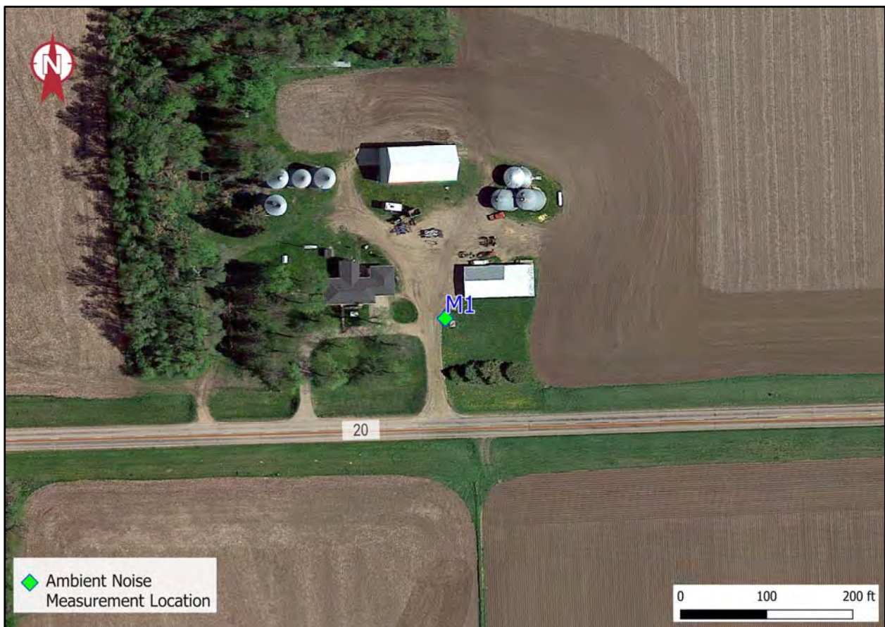
Figure 4-2. Measurement Location M1
