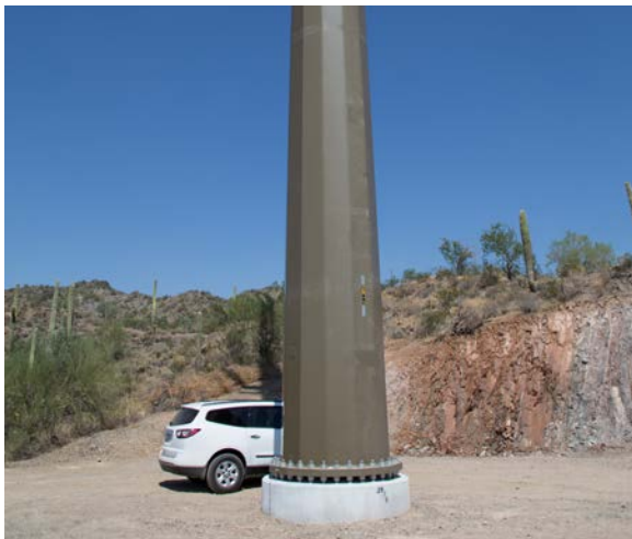
Figure 28 - Erected powder coated monopole
