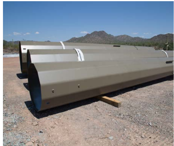
Figure 27 - Poles staged for placement
