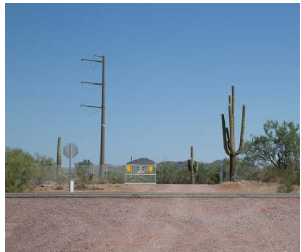
Figure 29 - Erected powder coated monopole
