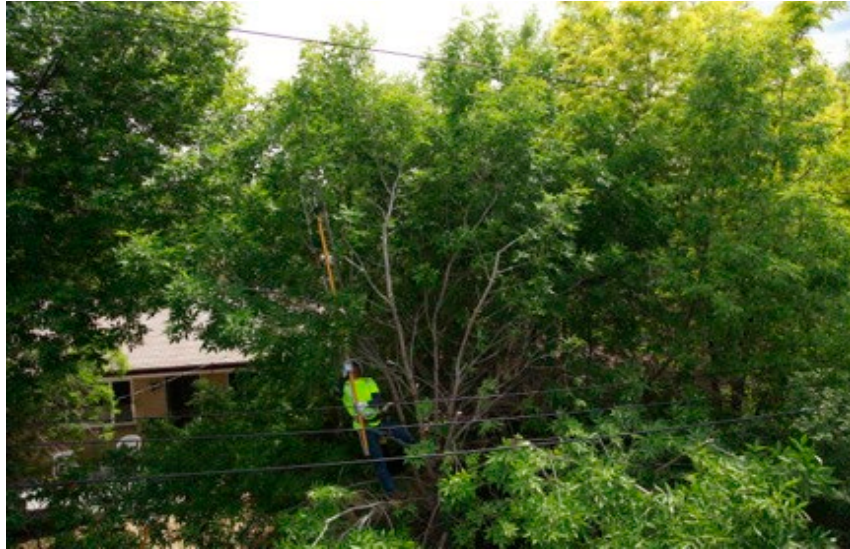
Figure 2-5 Example of Vegetation Management Function (Tree and Powerlines)
