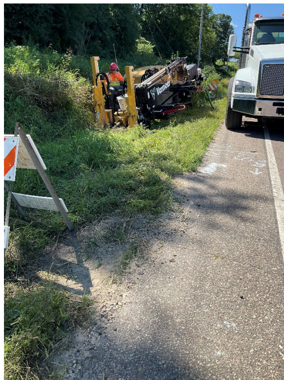
Figure 2-11 Directional Boring Operation Begins
