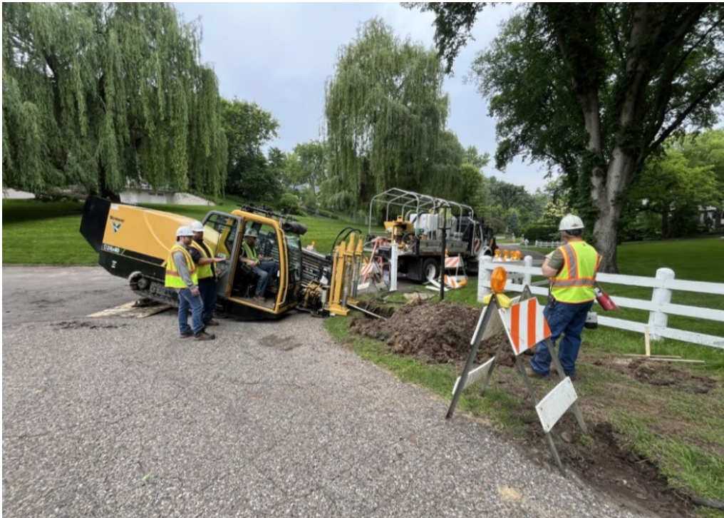
Figure 2-12 Directional Boring Operation Process
