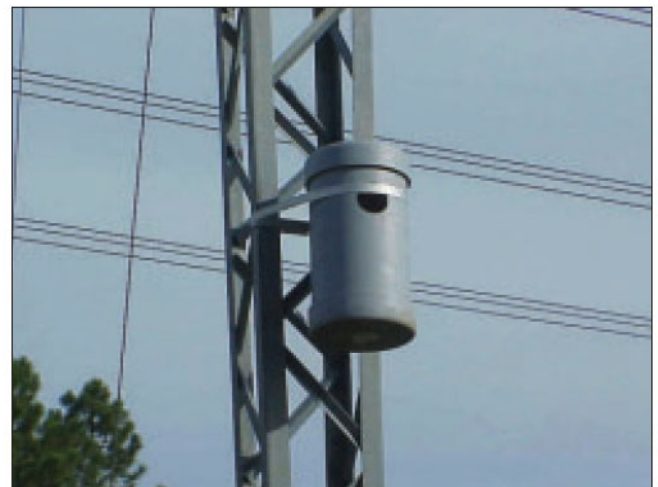
FIGURE 6.20 Kestrel nesting tube (46-cm [18-in] length) installed on transmission tower in Georgia.
