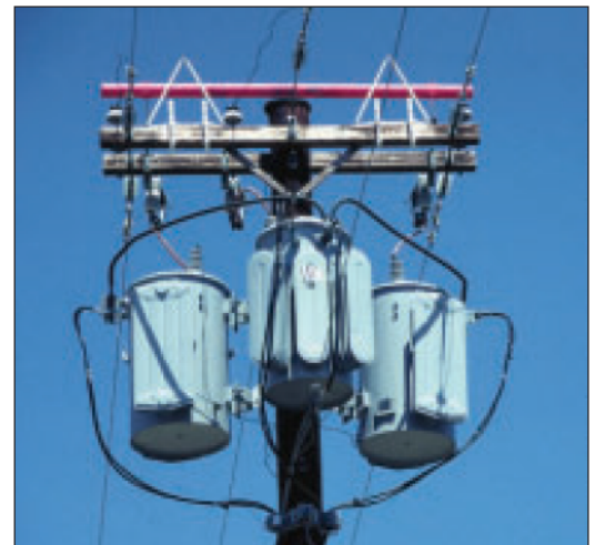
FIGURE 6.24: A pipe mounted above the conductors can be used as a nest discourager on distribution poles with insulators mounted on the crossarm. The use of triangles is cautioned against, as they may aid in the accumulation of nesting material. This design may pose an electrocution risk if exposed equipment and conductors are not covered or adequately spaced.
