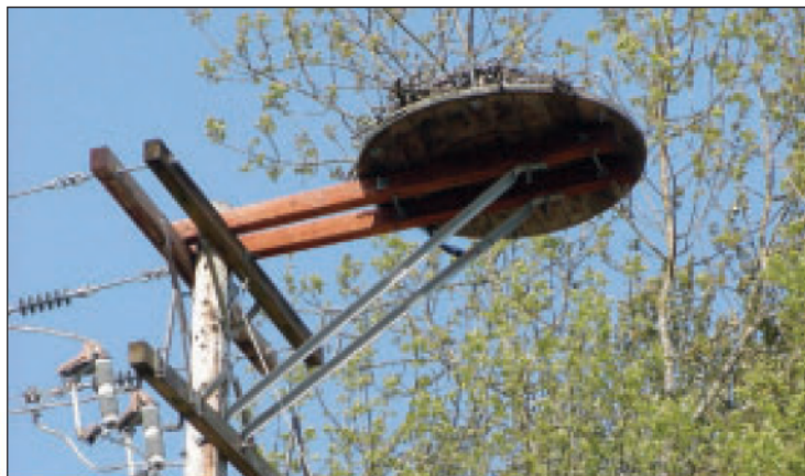
FIGURE 6.10: Osprey nest platform design developed by Portland General Electric. The platform is constructed from the end of a 1.5-meter (m) (5-foot [ft]) diameter wooden cable spool with coated cable along the edge to contain nest material. Utilities should ensure energized parts and equipment below the nest are covered to prevent electrocution of birds or outages from nest material. Consumer's Power, Inc. retrofitted this pole to their avian-safe standards.
