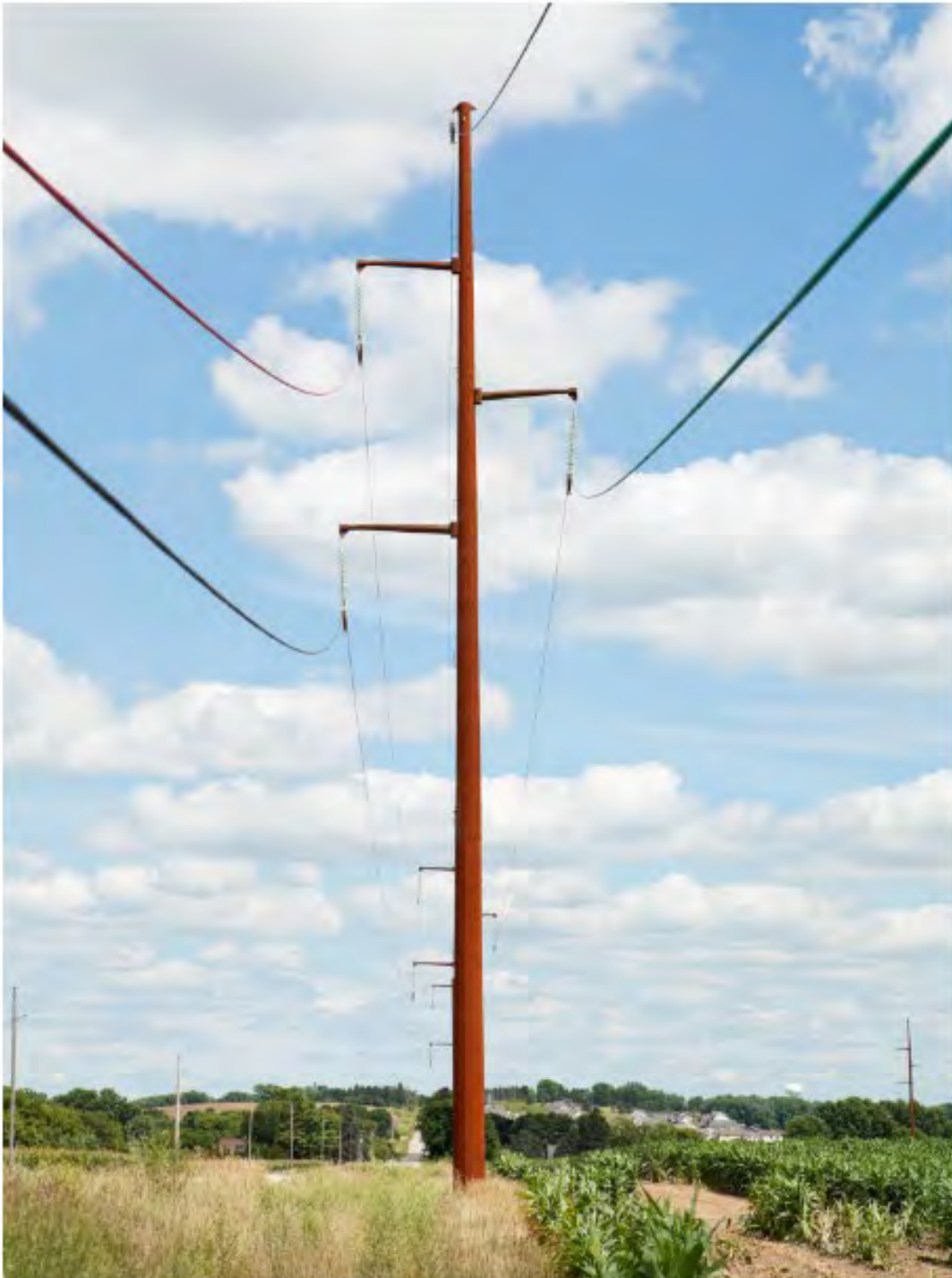
Figure 2-4. Photo of Typical 161-kV Transmission Structure
