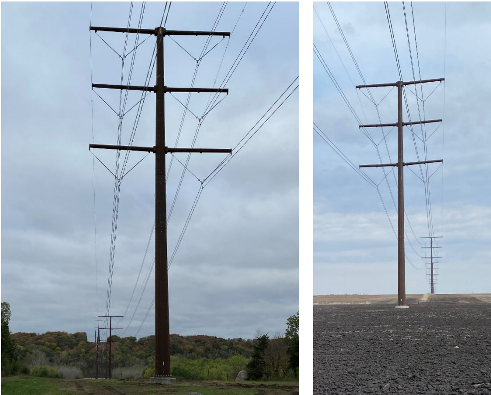
Figure 3-1 Example Double-Circuit, Monopole 345 kV Structures with V-String Insulators
