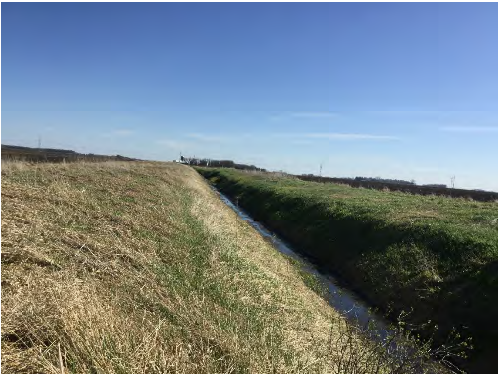
Photograph 8 (South): An overview of SA053.
