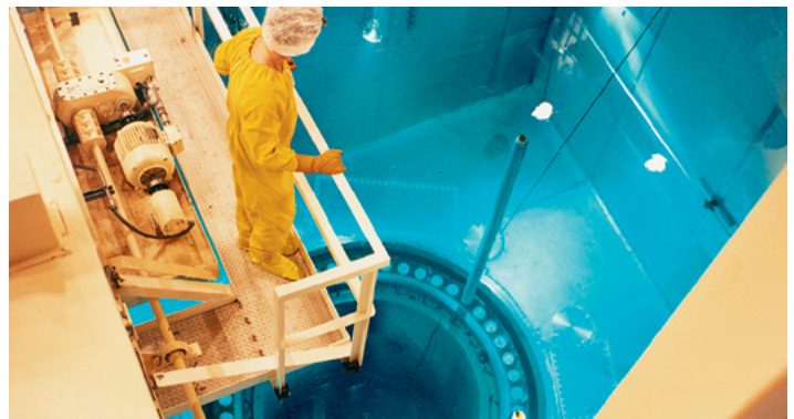
Used fuel at nuclear energy facilities is cooled in secure steel-lined concrete pools filled with water.
