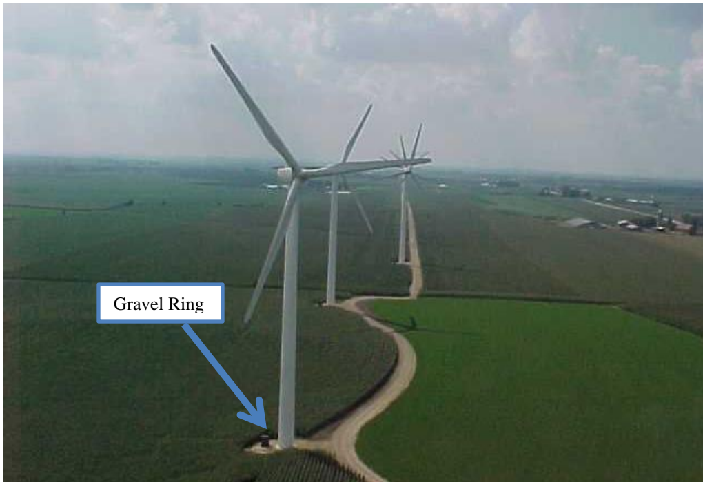
Figure 6: Gravel Rings and Access Roads
