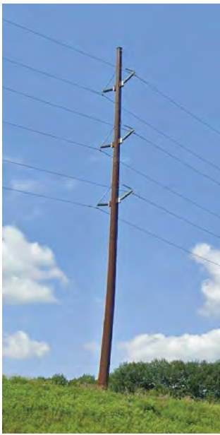
161/69 kV Steel Double-Circuit Monopole Structure
