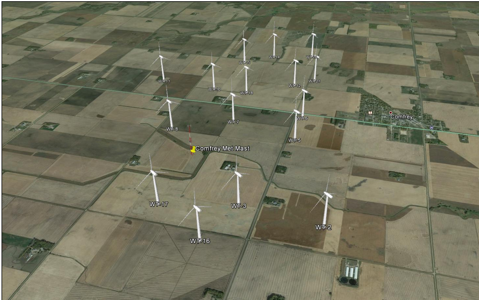
Figure 2. Comfrey wind farm detail 1, Vestas layouts and met mast location source Google Earth.
