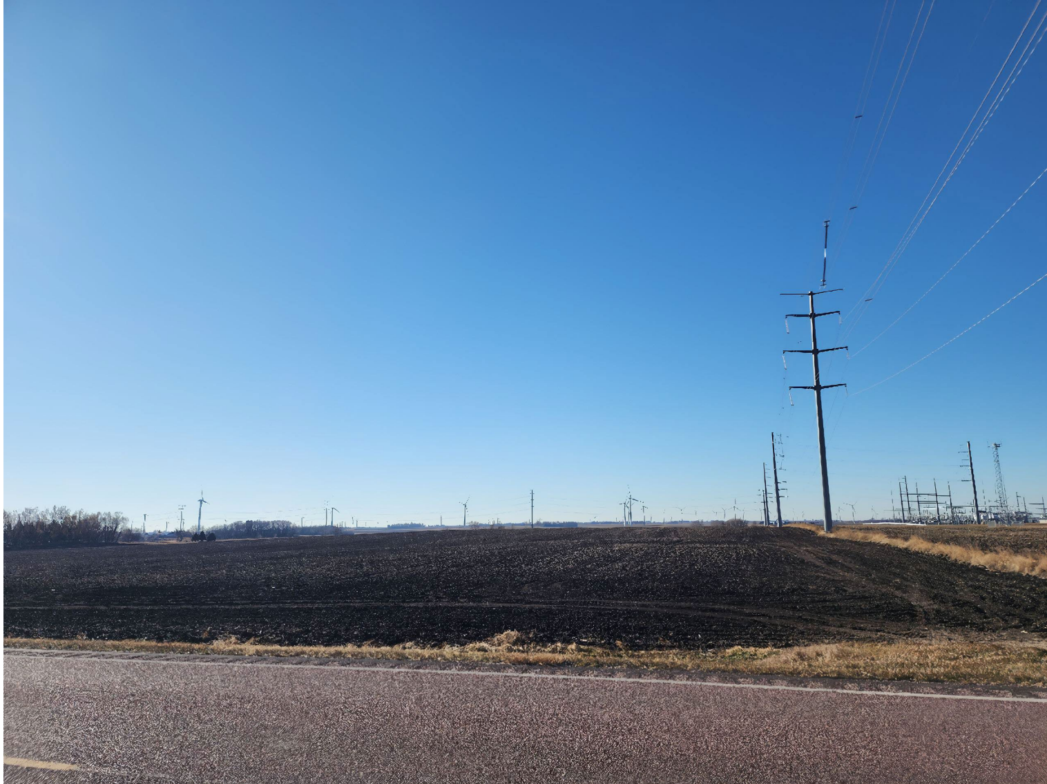
Figure 5.2.1-5: McCall Avenue Looking West – Existing View
