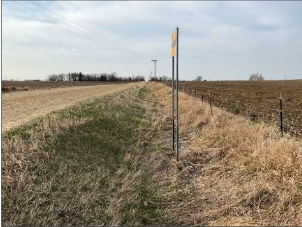
Photo 4.2-1. Overview of Area 2, facing south.
